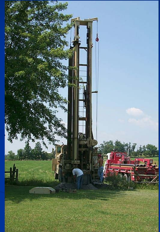
Drilling a new residential well
