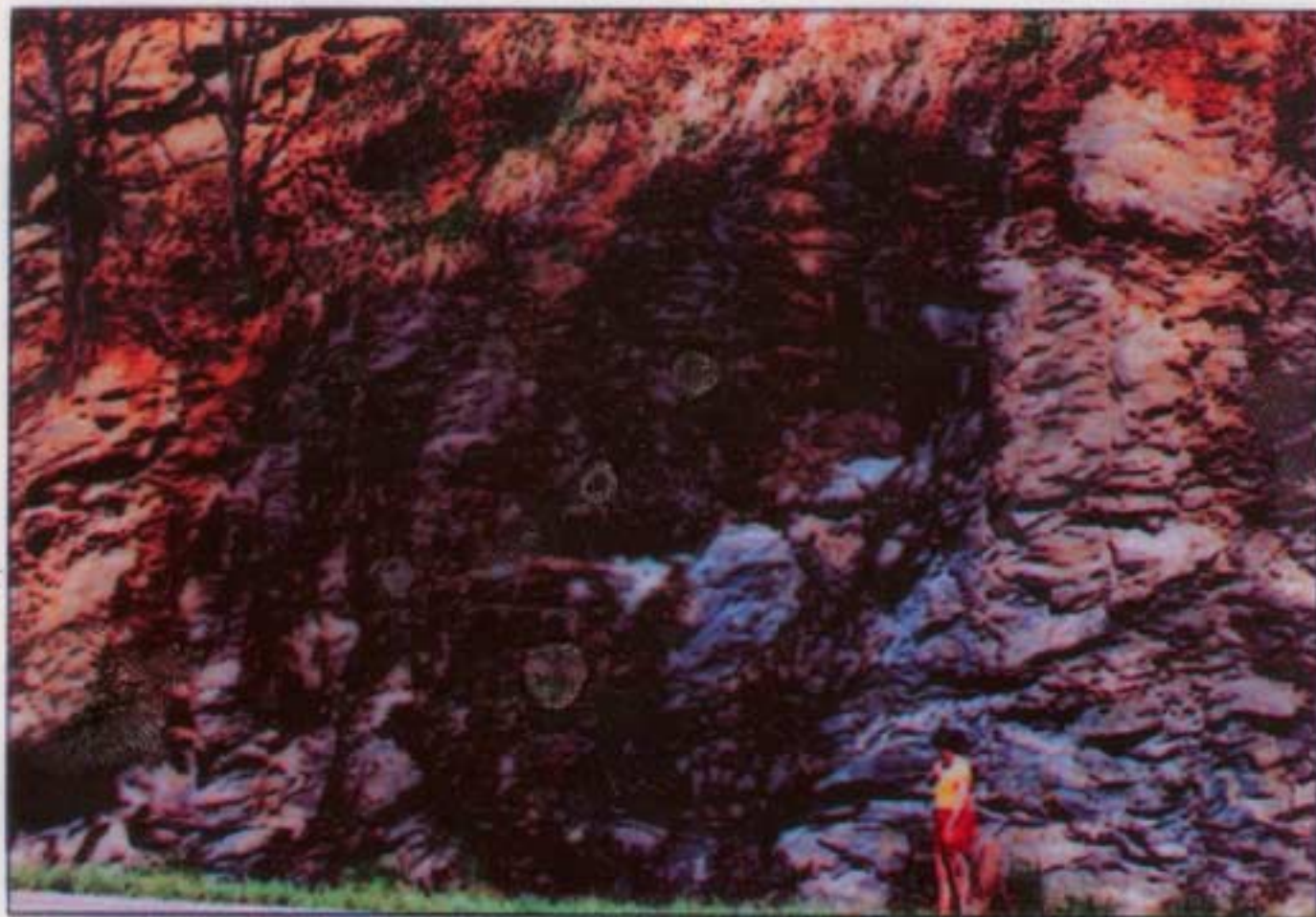
Figure 86. In crystalline rocks, water moves through fractures. The dark spot in the photograph of this roadcut shows where water issues at the rock face from part of a nearly horizontal fracture. The water has first moved downward through vertical fractures, then moves laterally to its point of discharge. The surrounding, lighter colored rock is dry.
